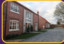
Project by Keigar Homes Ltd
